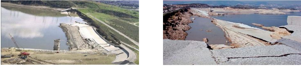
Figure 1 : Break of the San Fernando Dam
